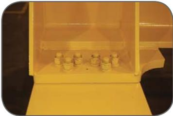
Standard bolted girder connection plates
